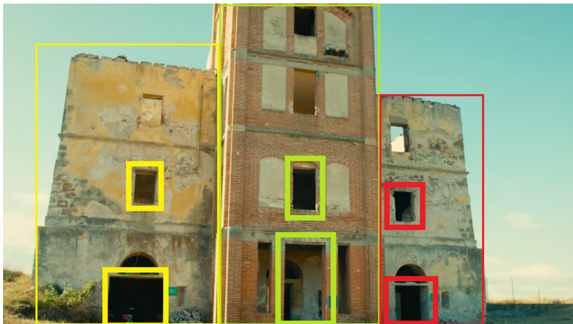
Figure 31. Three possibilities for wall inspection, the one to be inspected will be decided during the competition days (Photo credit: euRathlon).
