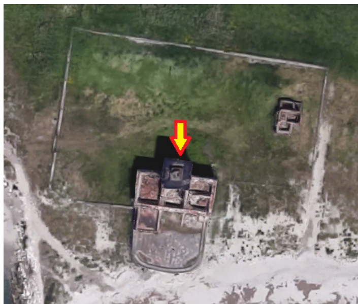
Figure 32. Example of designation of the wall to be inspected (Photo credit: euRathlon).
