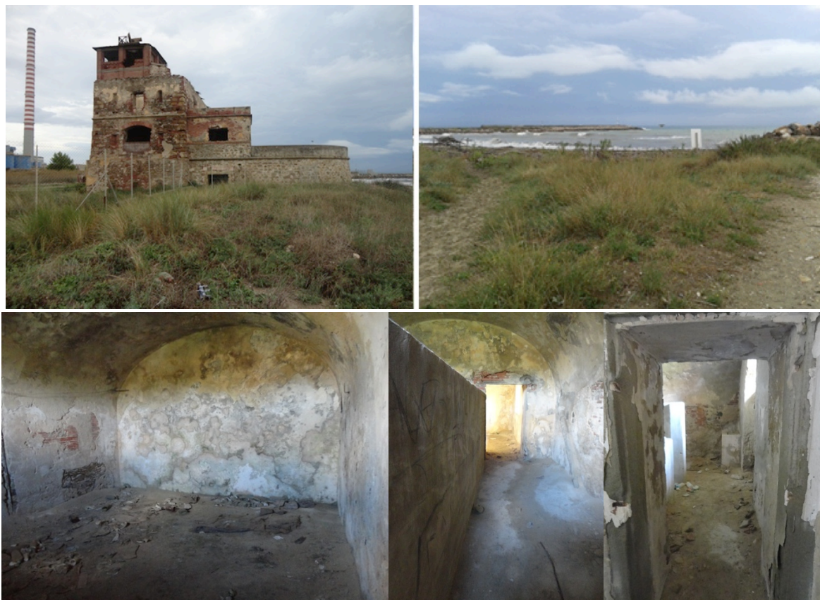
Figure 3. Building, shoreline and interior. (Photo: euRathlon).
