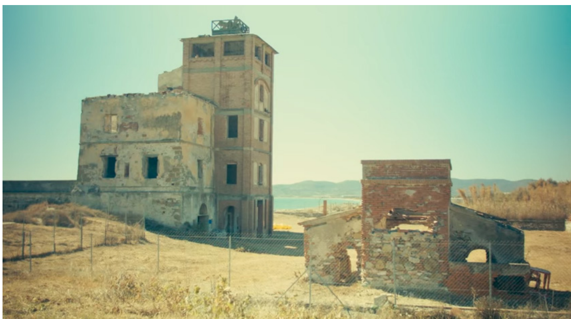
Figure 30. Damaged building to be inspected (Photo credit: euRathlon)
